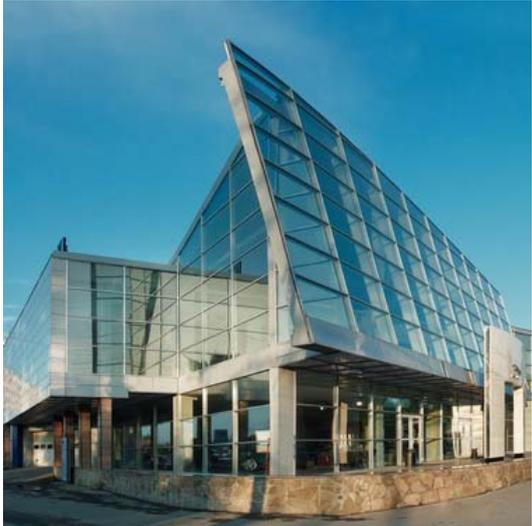
Building envelopes using the energy efficient FOPPE RP50+SI facade system
